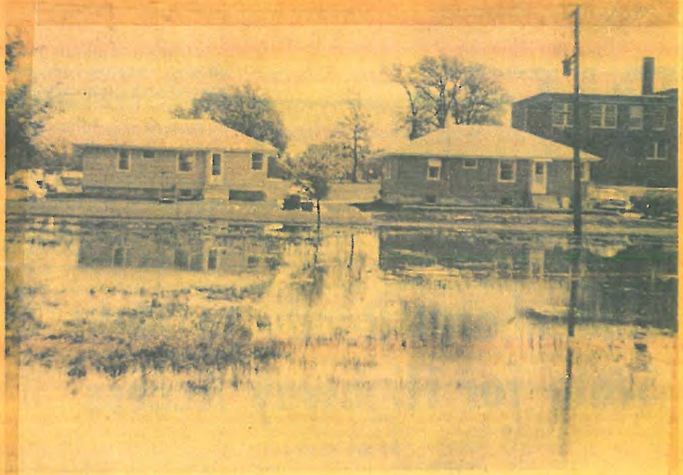
EDINA FLOOD ZONE located in the Morningside area features for to five foot deep lakes of water throughout the summer with floods after each storm. The large building is Morningside Elementary School.
