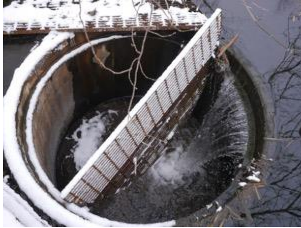
Figure 12. The outlet structure that transports water from the TIA to Weber Pond via the stormsewer system
