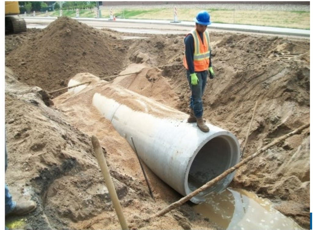
Storm drain installation
