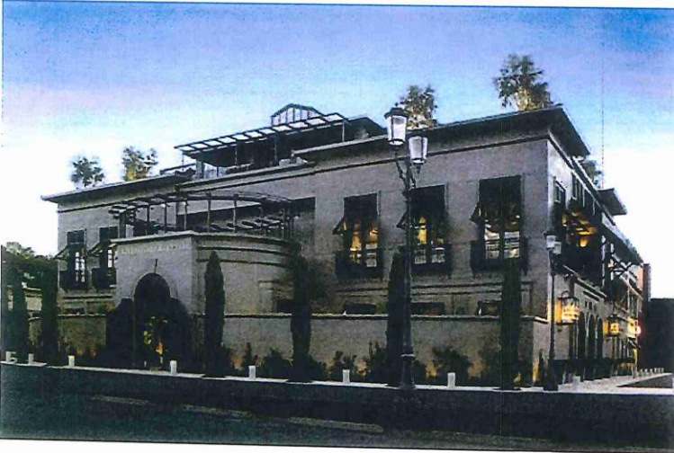
Atlanta Restoration Hardware With 8 foot high wall along public street
