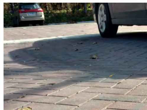
Permeable parking lot bays
