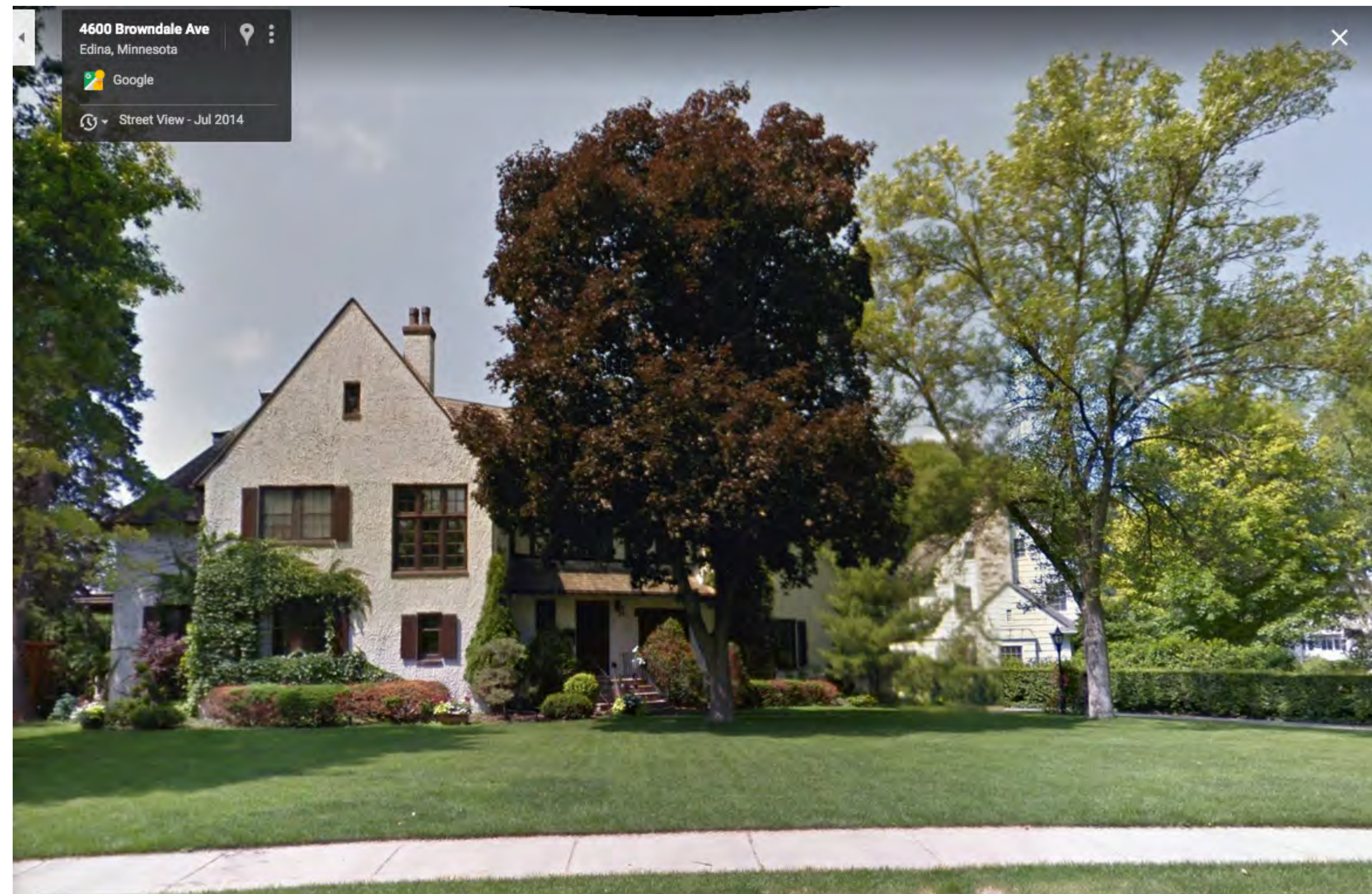
Street Facade showing main gable fenestration
