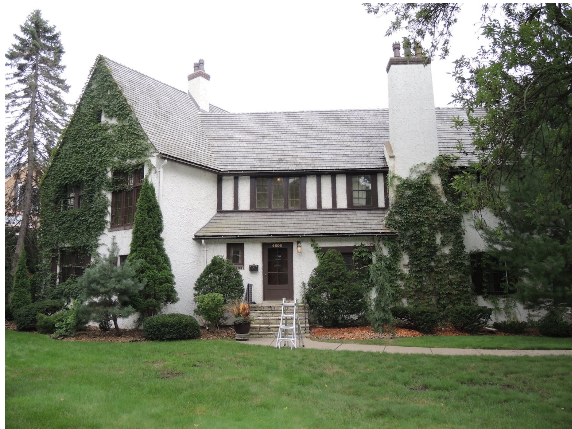
Close up of Existing Entry
