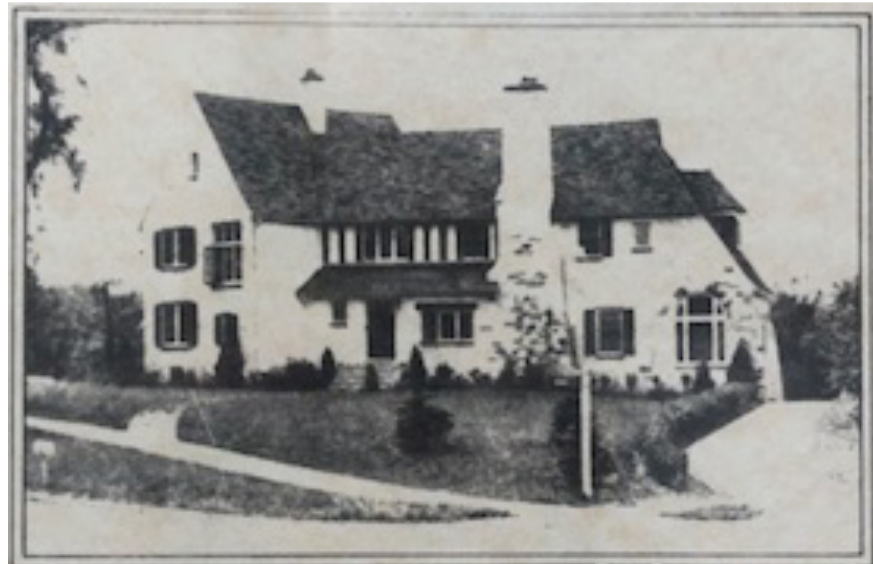
Street Facade soon after construction
