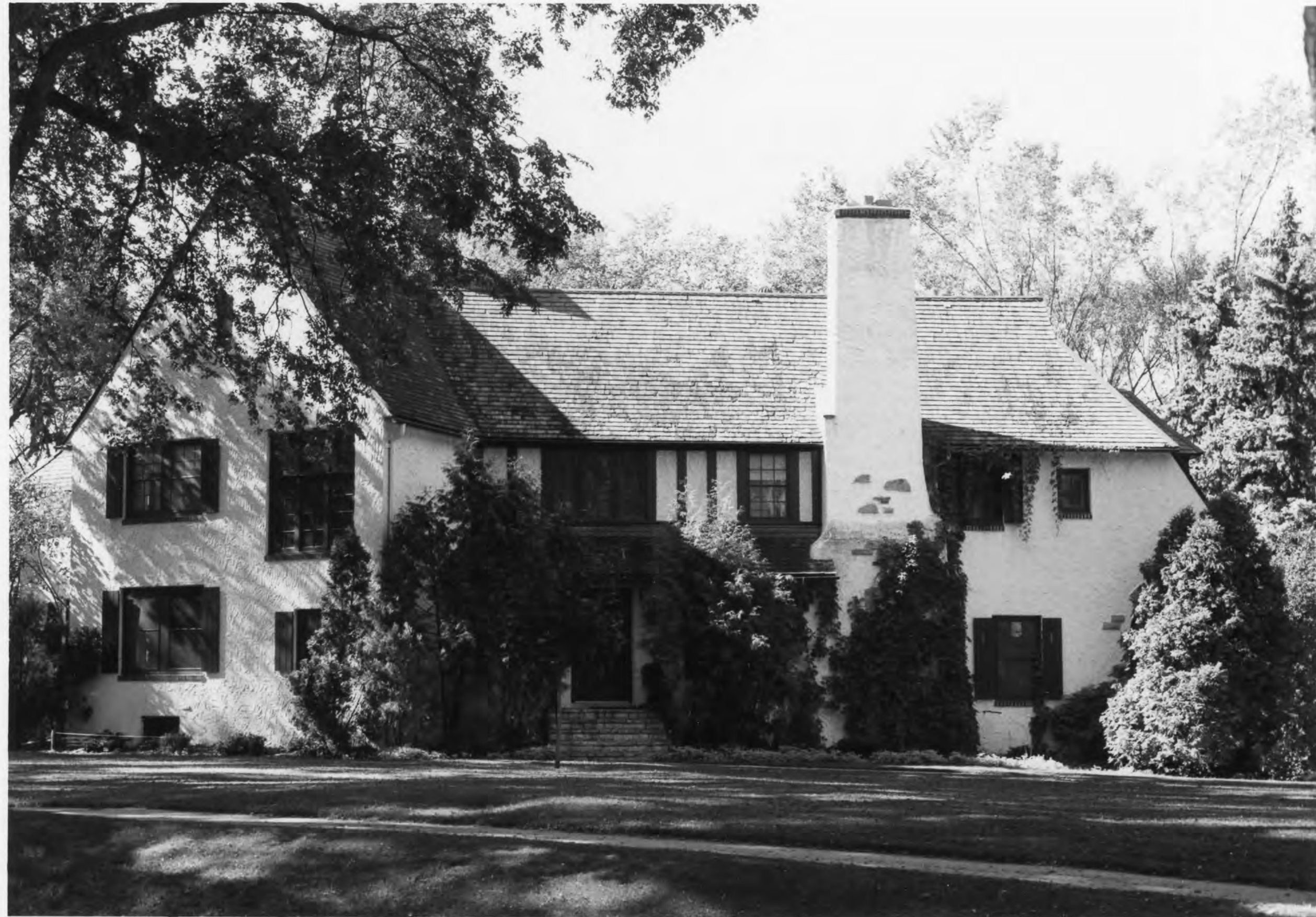
Street Facade showing main gable fenestration
