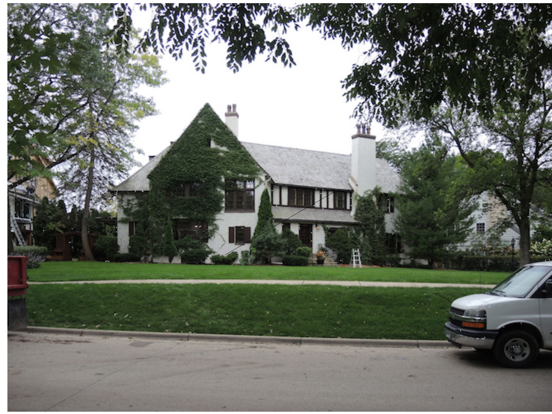
Existing Street Facade
